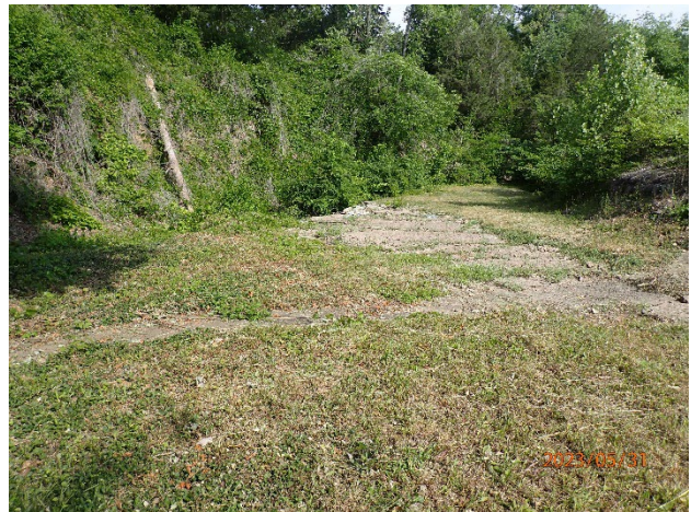
Principal spillway channel- looking downstream
