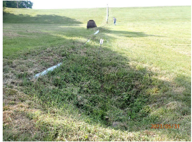
Siphon system and historic depression to monitor for change
