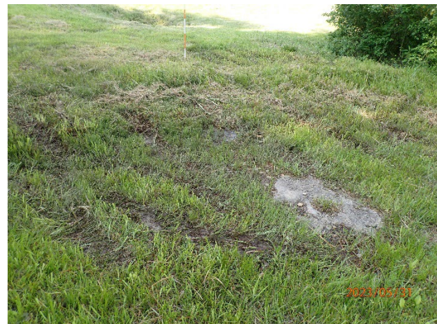
Seepage area near right groin
