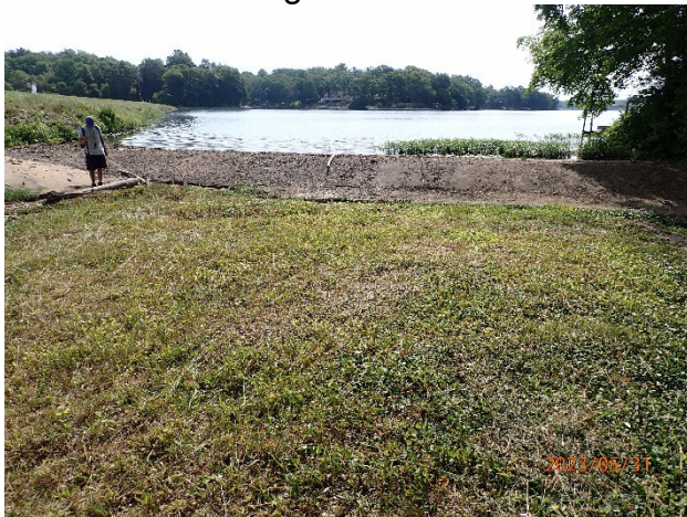
Principal spillway channel- looking upstream
