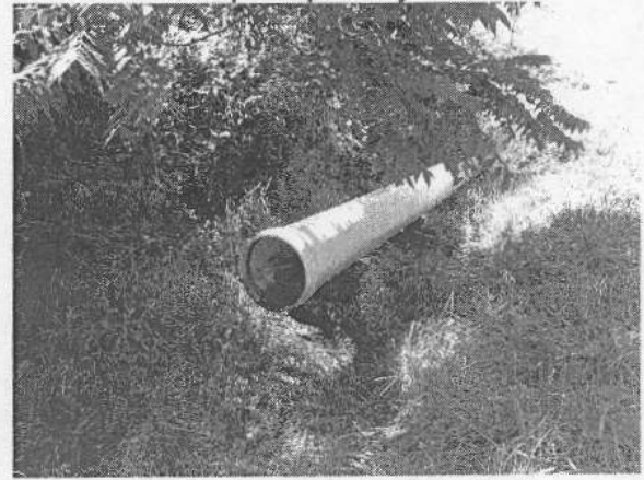
Embankment drain outlet
