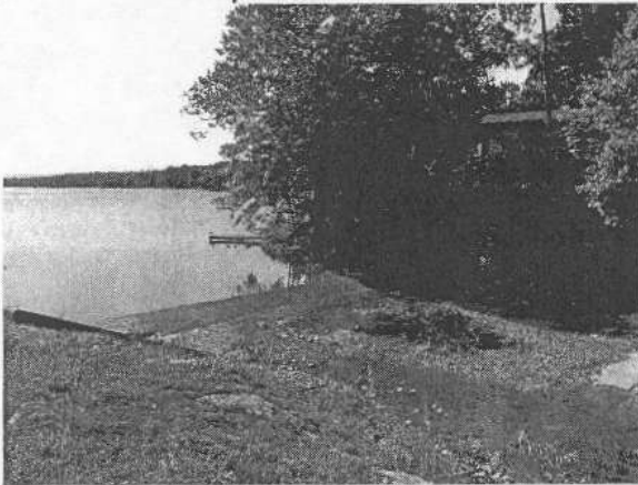
Principal spillway inlet
