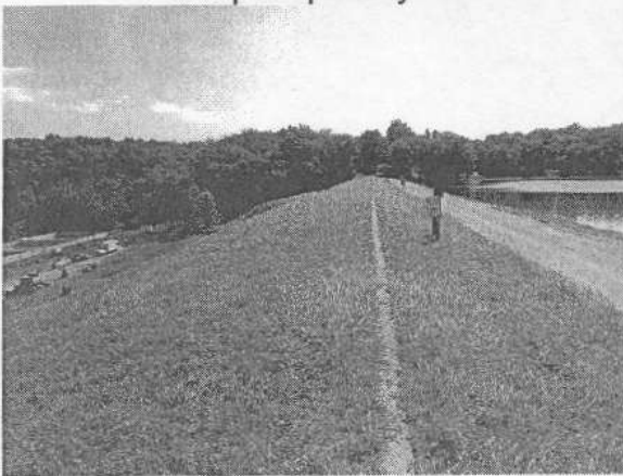
Crest of dam
